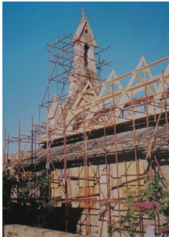
Resurrection: the new roof trusses and associated structure are in place as work advances on restoring the Church: 1988 July
